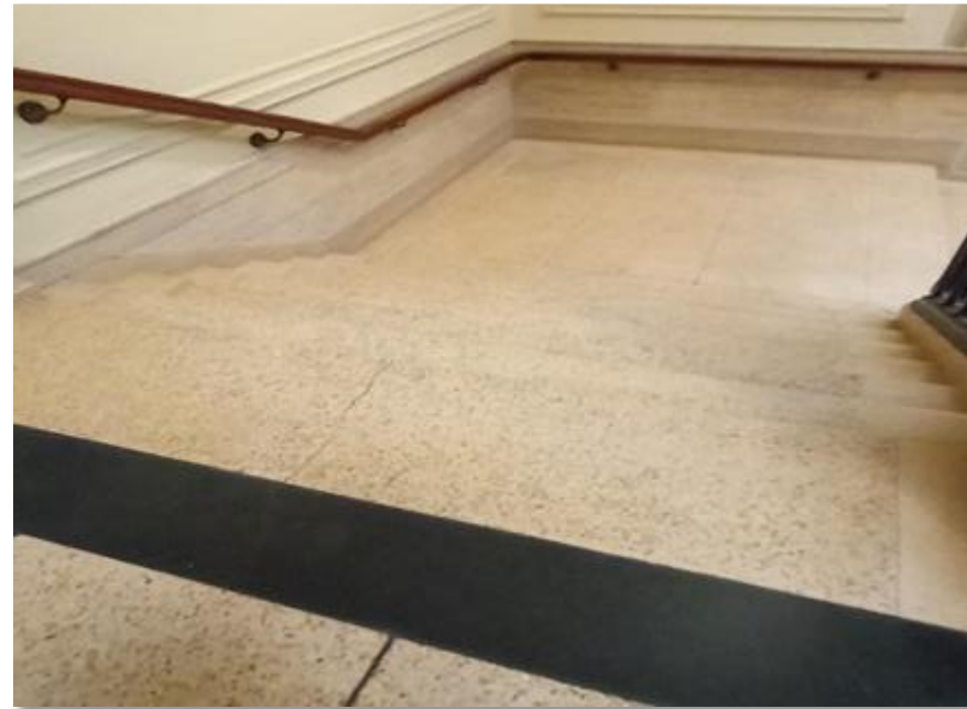
Gallery stairs down to Ground Floor with handrail.
