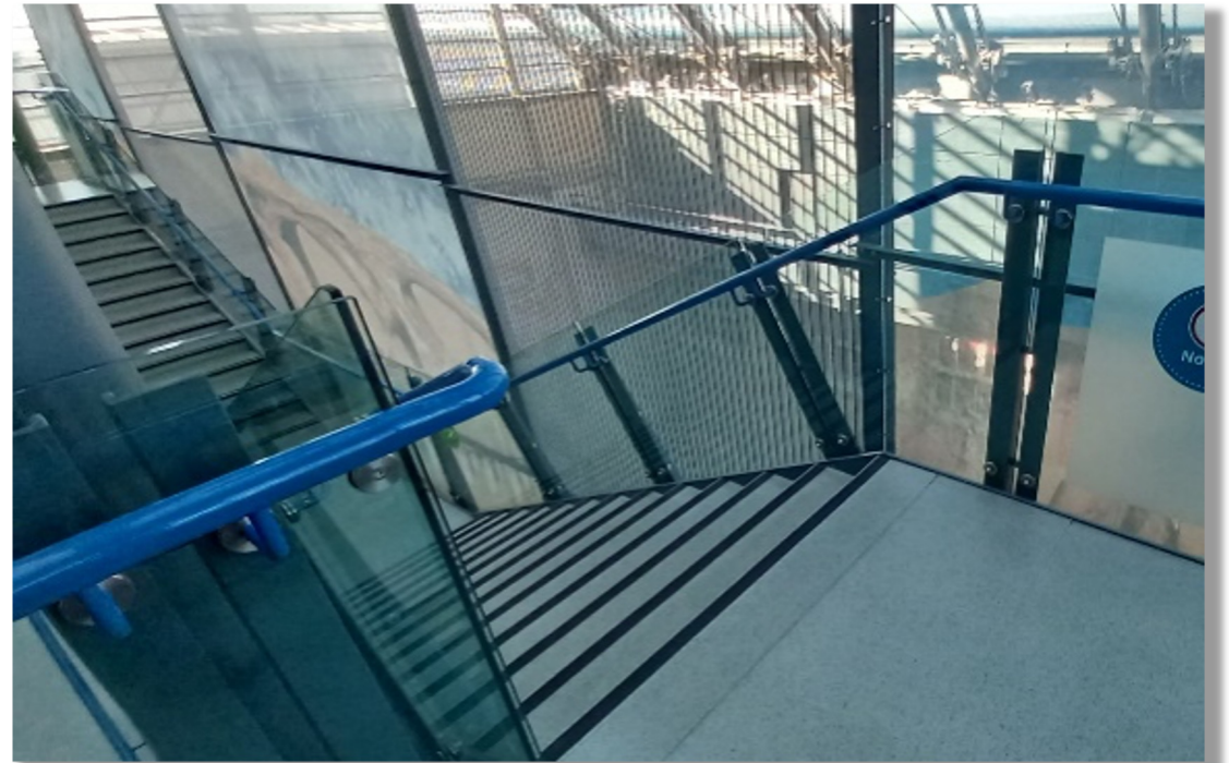
Stairs with blue handrail and glass walls
