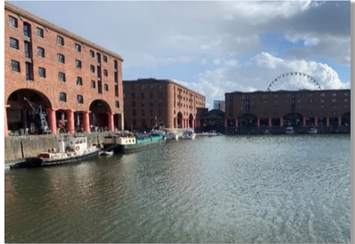
View of the Albert Dock from the picnic area with the Dock basin in the foreground
