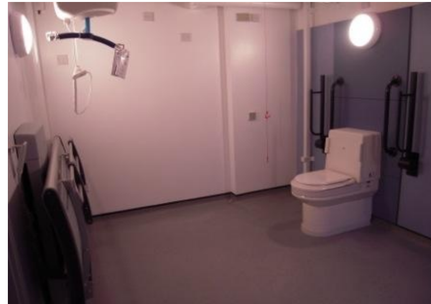
Changing places toilet
