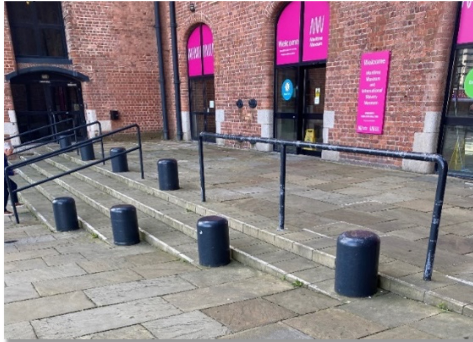
Concrete steps, black handrails and black bollards located outside the main entrance
