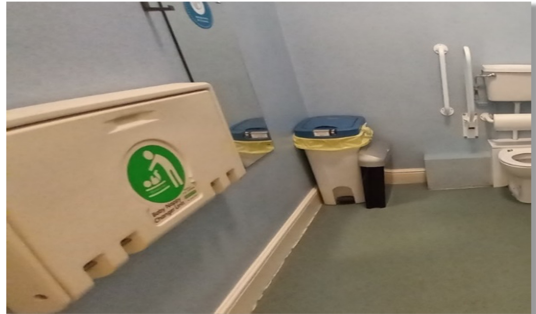
The accessible toilet with fixed height baby changing unit, pull down and vertical grab rails
