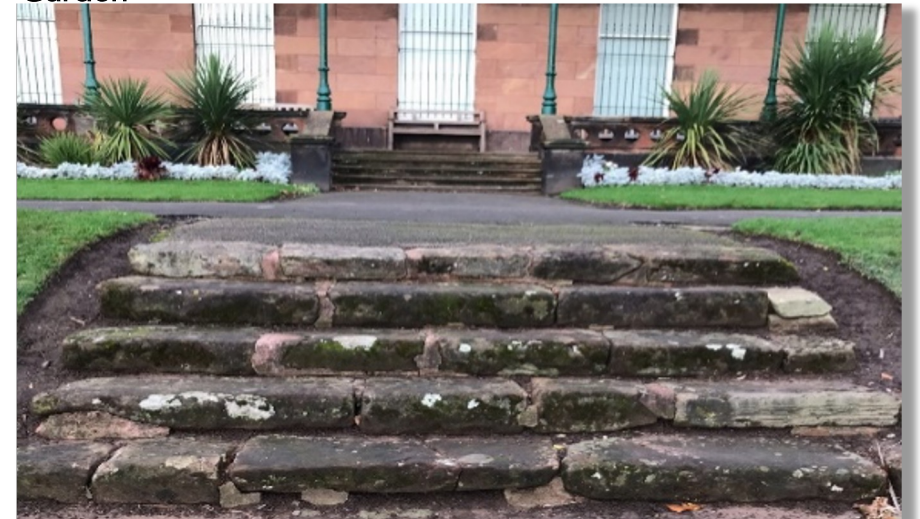
Stone slab steps located in the Hillsborough Memorial Rose Garden. These can be uneven.
