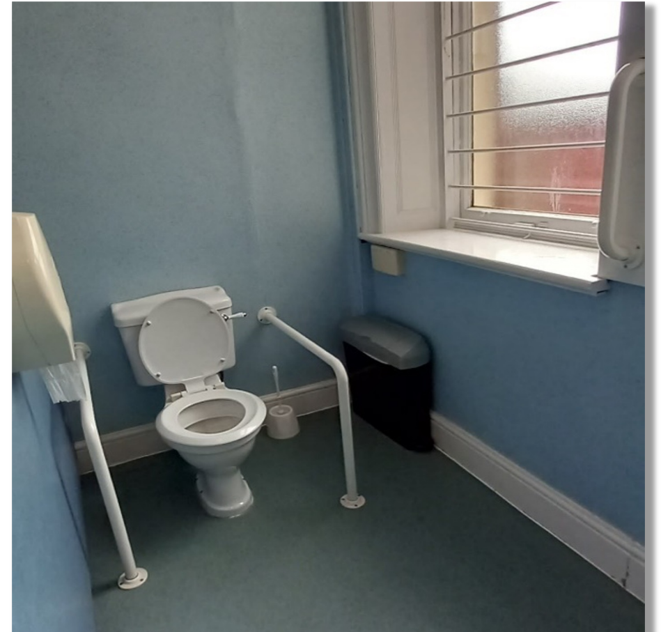
The Ambulant Mobility toilet. Includes fixed height toilet, two freestanding horizontal grab rails, bin and toilet roll dispenser
